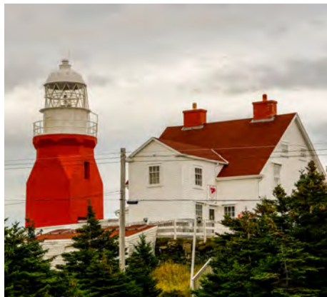
Long Point Lighthouse
